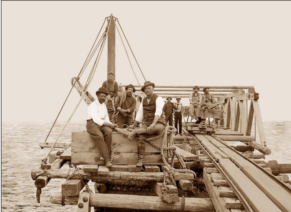
Figure 28: Ronksville pier, with Ronk brothers (foreground) and workers (background). Truss system is present rather than the building that appears in Figure 27. Railcar and rail system readily apparent. Date of photo unknown. Photo submitted by Jonathan Ronk.
