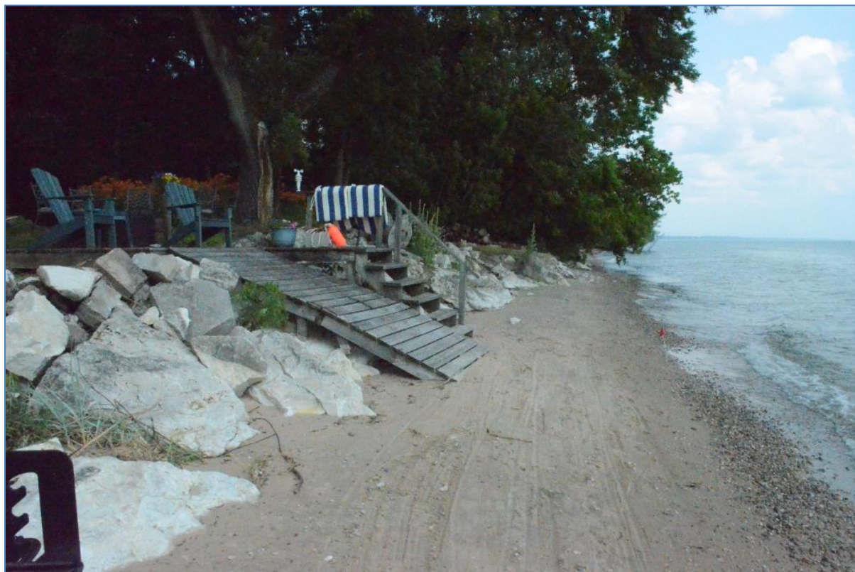
Figure 7: Modifications to the current high water escarpment in the form of rip-rap (foreground). Note narrowness of beach and pebble concentrations at surf line. Photo taken looking north from 6878 Jay Beach Road South.
