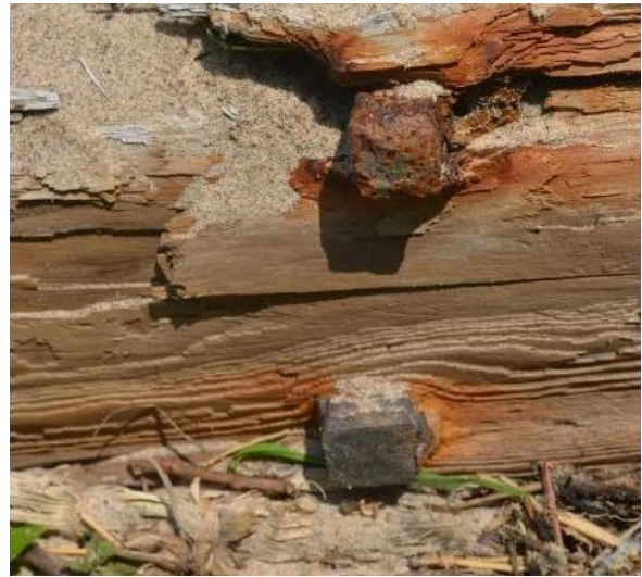
Figure 33: Detail of drift pins on exposed pier fragment.
