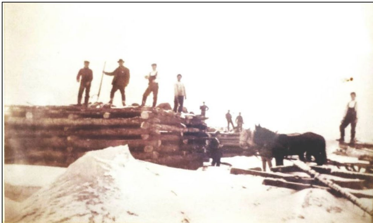
Figure 36: Pier cribs and workers, possibly recording construction of an iteration of the Ronksville pier. Photo provided by the Lake Church Tavern.
