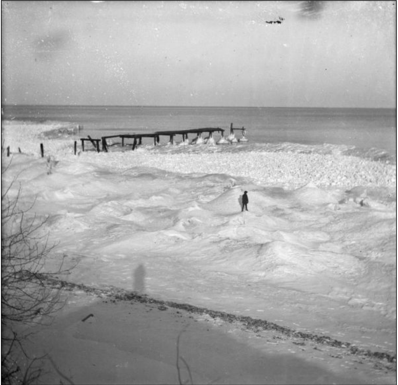
Figure 38: Photograph by Harry Dankoler, ca. 1905, showing damage from storm and ice to a Lake Michigan pier in Door County, Wisconsin. WHS Image ID 69430.
